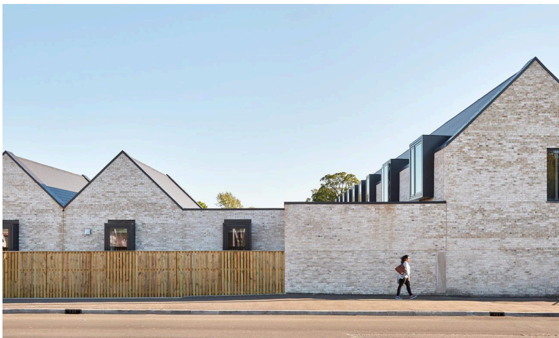
Figura 17 – Vista externa do Ronald Mcdonald House
