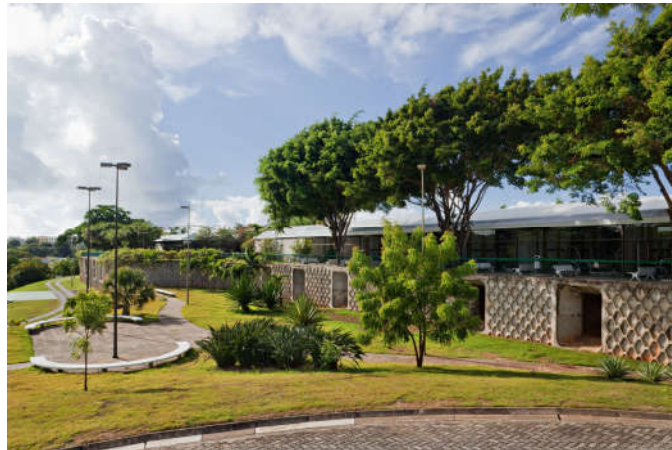
Figura 11: Fachada Principal – Hospital Sarah Kubitschek Salvador
